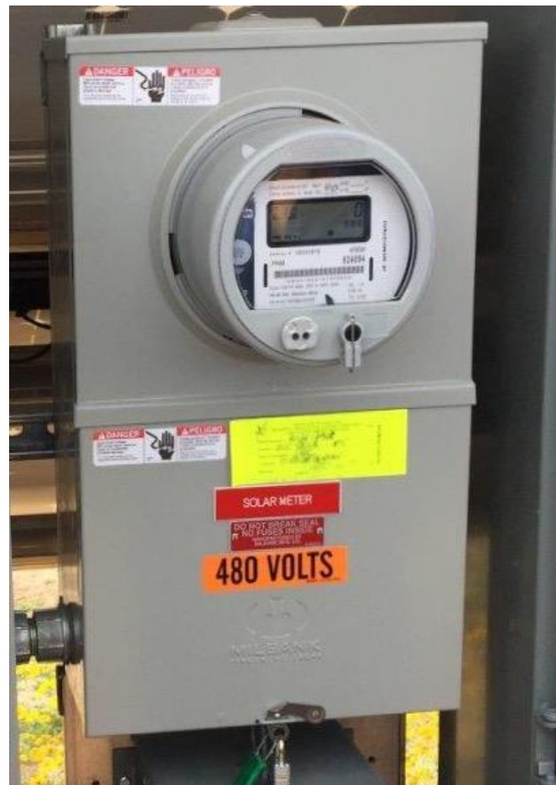
Properly Connected Meter
